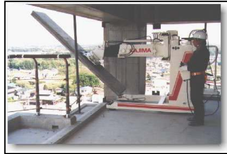
Figure I.32: Robot de construction
